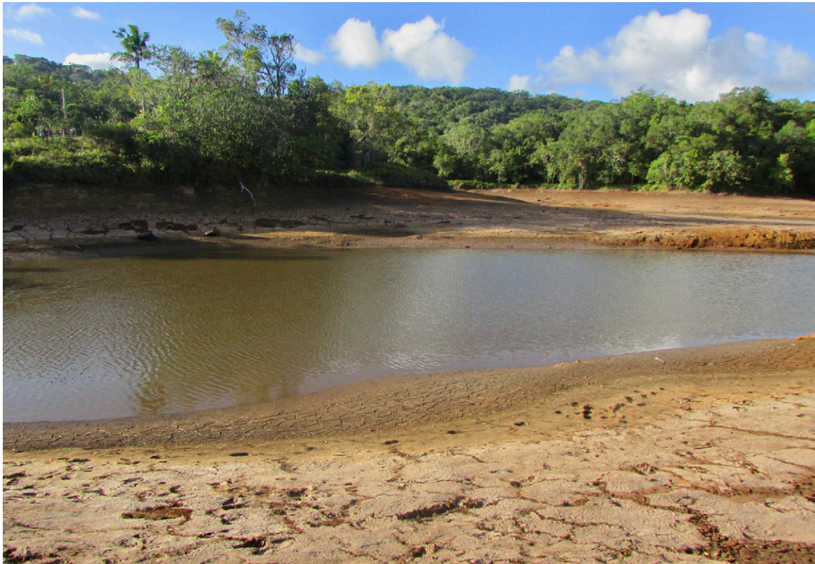
The Ngerikill River and Ngerimel Dam system provides the majority of the public water supply for Koror and Babeldaob. The drought of 2016 left water levels in Ngerimel Reservoir (pictured) dangerously low. Photo: Palau Public Utilities Corporation.
